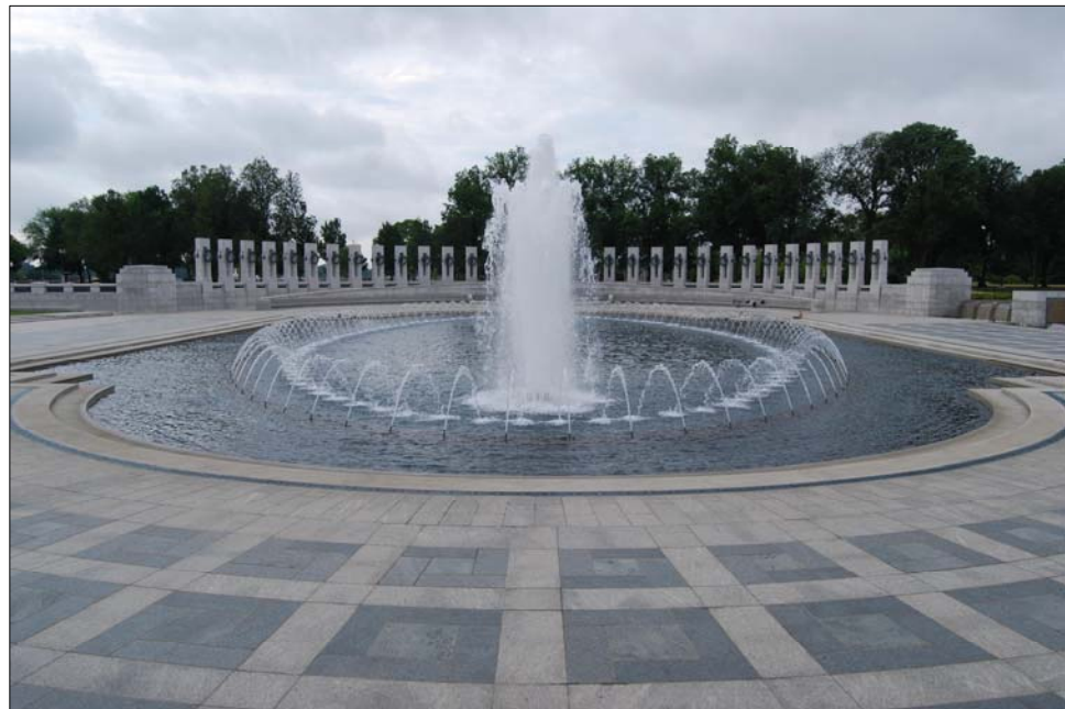
Granite paving patterns underscore the use of quality materials and add interest to large open areas.
